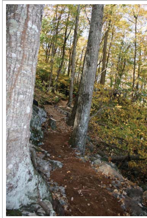
A new trail section is just completed at Rocky Knob Park. photo by Taylor Woolridge
